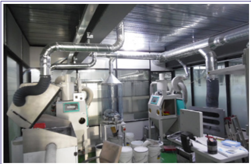
▲ Installation of local ventilation system and prevention facility
