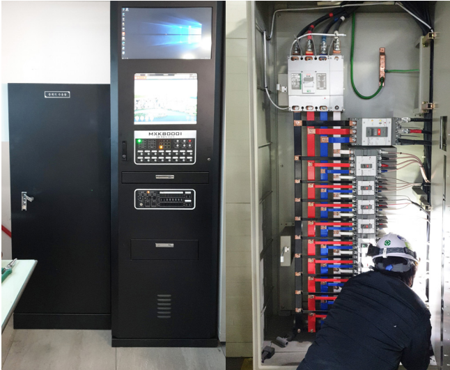
R-type Digital Fire Alarm Panel
